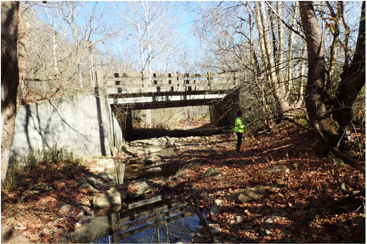
Typical upstream view.
