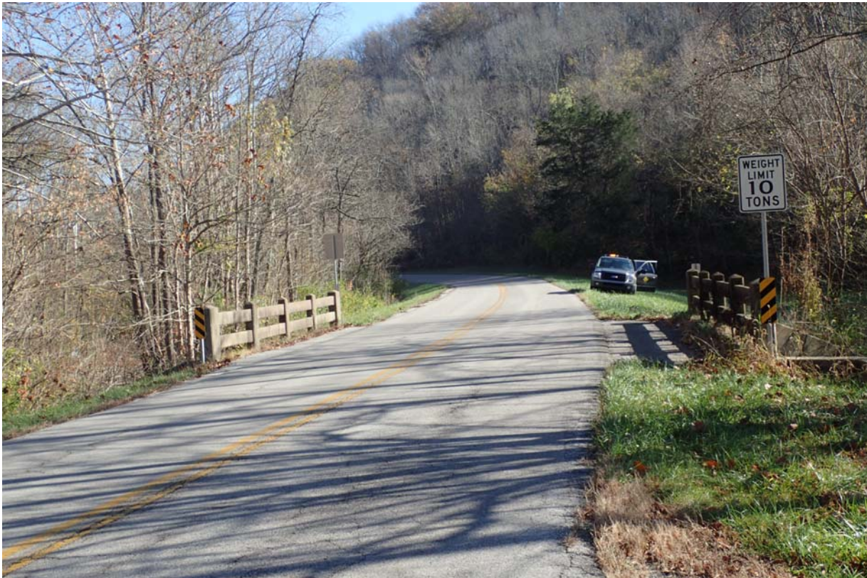
View of the 10 tons posting sign near abutment 1.
